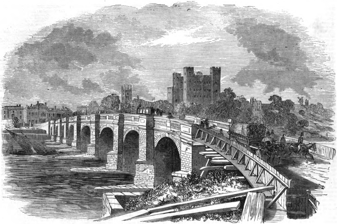
ROCHESTER OLD BRIDGE.
